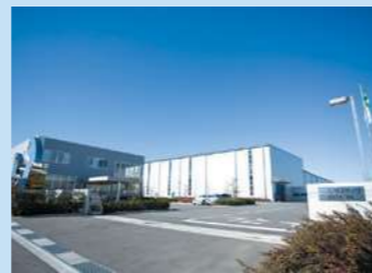
Main plant entrance and office
